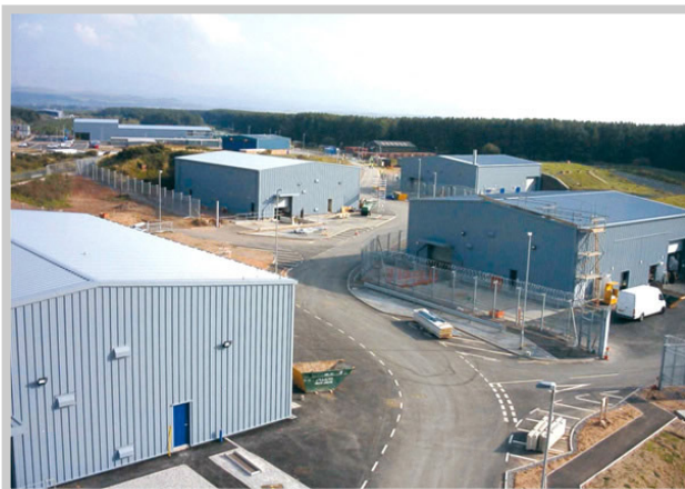
PCM decommissioning project
