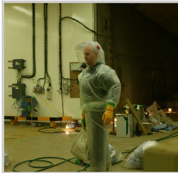
Decommissioning activities inside a PCM Magazine at LLWR Site
